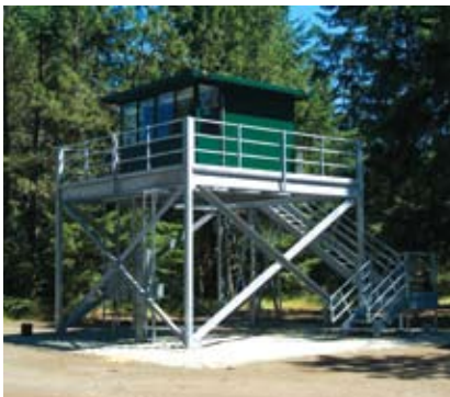
Tower at military installation gives guards visibility over a larger area than booth placed directly on the ground.
