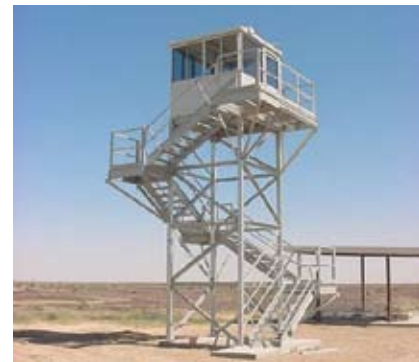
Tower placement on Federal Training Facility allows range master to view firing range and to see results from above without ground level obstructions.
