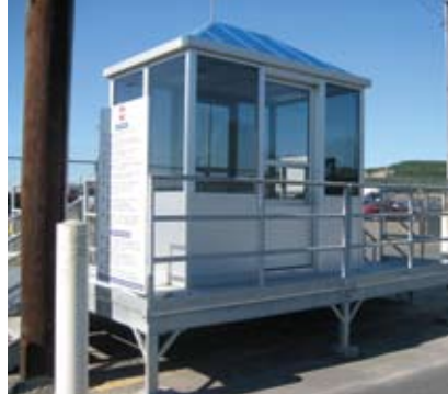
Parking lot security has increased viewing area from booth placed on special height platform.
