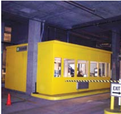
A custom painted exterior was added to make this combination modular garage office and cashier station easier for patrons to locate.
