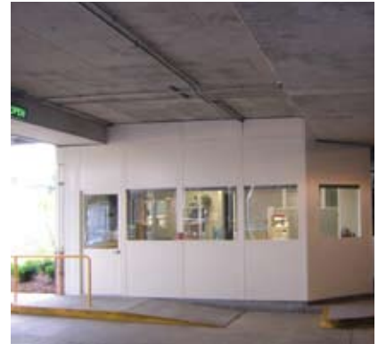
The modular panels used to construct the office inside this hospital parking garage were custom designed to fit under the existing ceiling structure.
