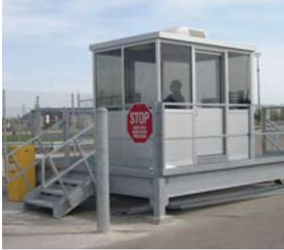
Platform position at entry/exit to distribution center allows guard to walk around for vehicle viewing and still have protection from the elements.
