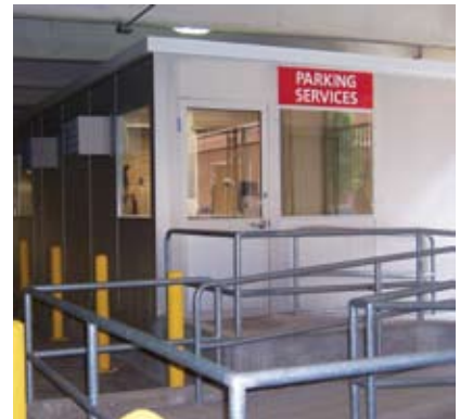
Ballistic rated walls were incorporated into this modular garage office to enhance security for personnel during off-peak hours of operation.
