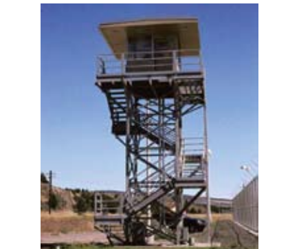
Guards at correctional facility needed elevated perimeter building for additional control.
