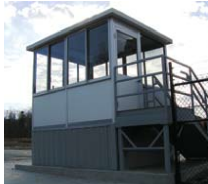
At the right height, facility guards can see inside trucks and other vehicles entering and leaving supply yard.
