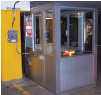
Modular construction enabled this parking booth to be assembled on-site deep within this parking garage where limited ceiling clearance prohibited the use of a preassembled booth.
